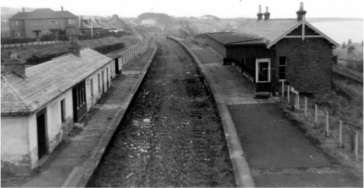
Largo Station, 1969, four years after closure to passengers. The indentations left by the railway sleepers can be seen imprinted in the ballast. When the line was first opened on 1 st February 1857, Largo Station only had a single platform, on the left, with a simple station building. In 1894 the passing loop and second platform were added, together with a more substantial building and canopy on the westbound platform. The goods yard was to the left, behind the original station building. Largo remained a passing place for trains until closure on 6 th September 1965.
