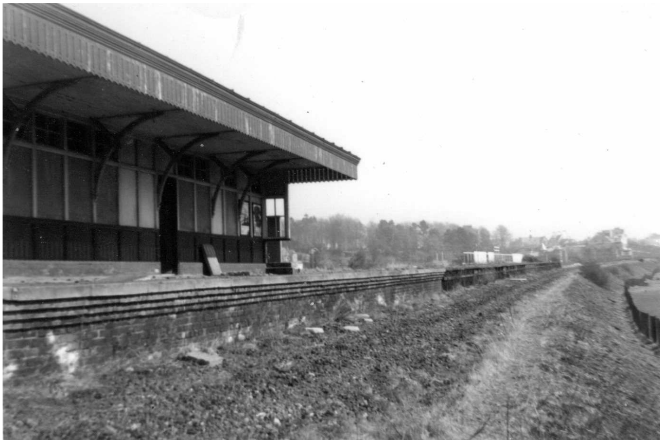
Looking east from Lundin Links Station towards Largo in 1969. Most of the platform fencing has been pulled down, but the frame for the station sign is still standing. After demolition of the station the land was bought by the golf course and the embankment swept away, allowing the two divided parts of the course to be united.
